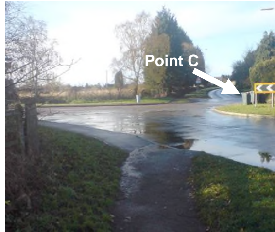
Looking west along Clophill Road towards the road junction and point C (behind bins and chevrons).
