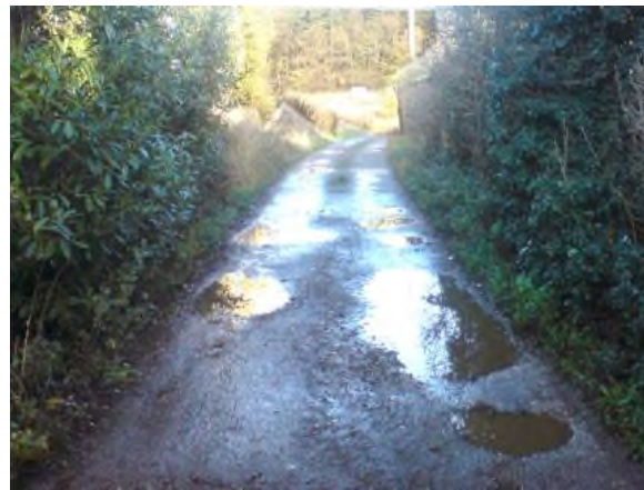
Looking north along Bridleway No. 24.
